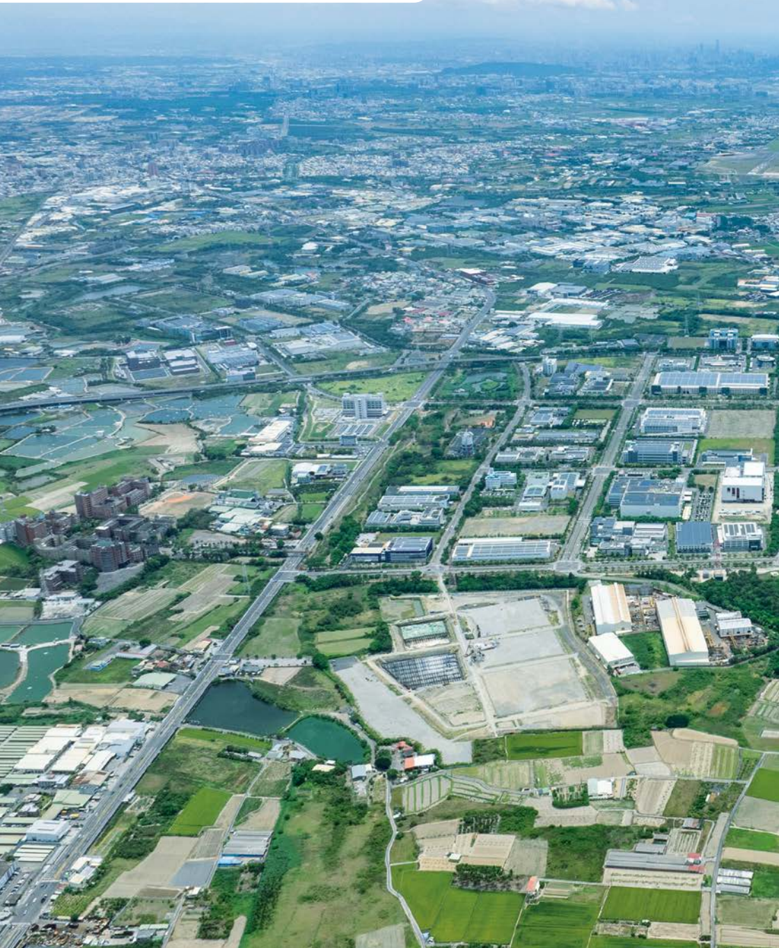
Full view of Kaohsiung Science Park
